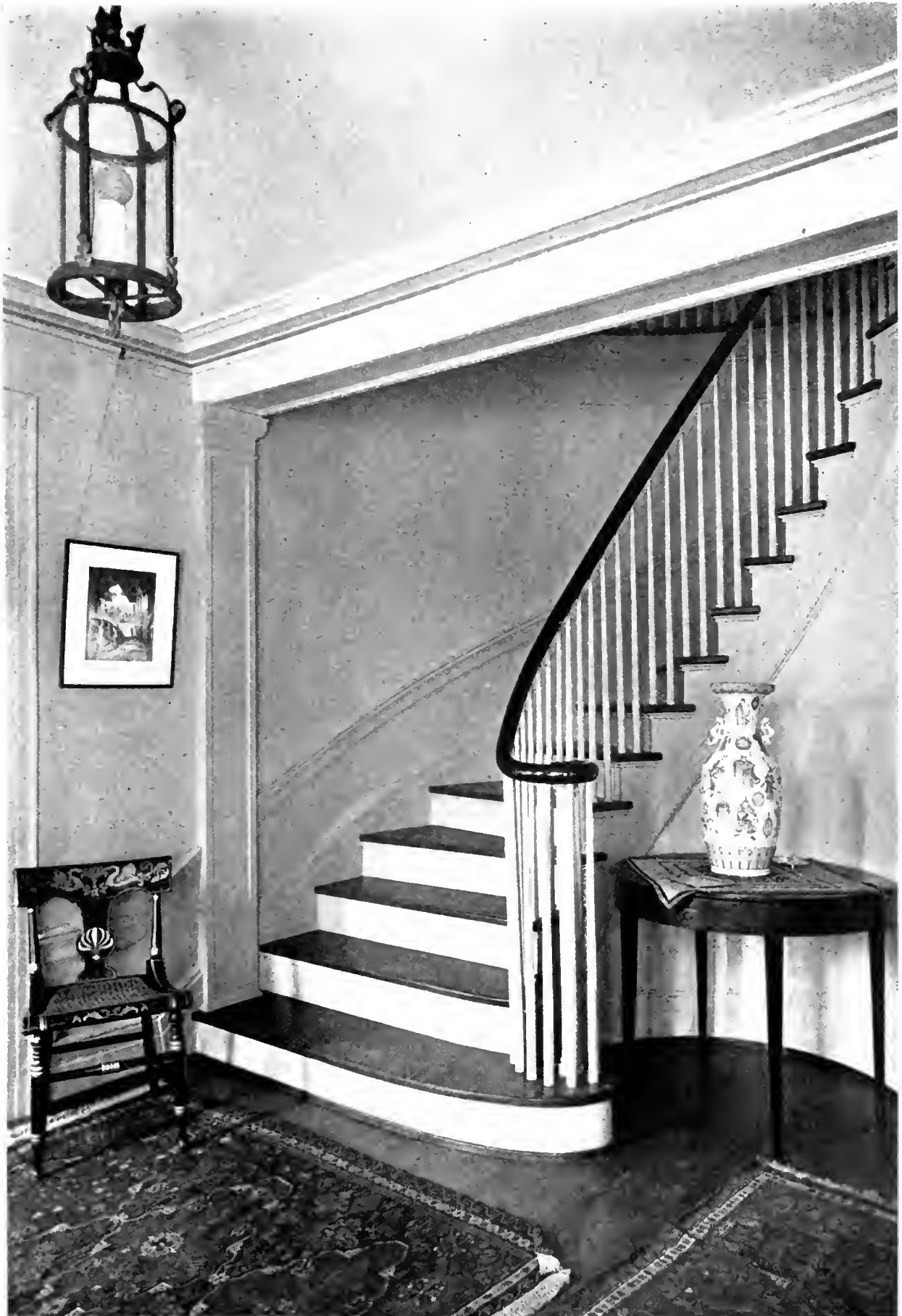
STAIRWAY HOUSE OF MR. JOHN W. GRIFFIN, FIELDSTON, N. Y.
